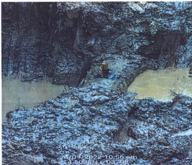
FIG 1: Installed 2 1/2" valve on the facility
