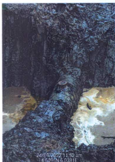
FIG 2-3: Incident Facility repaired and Aqua wrapped
