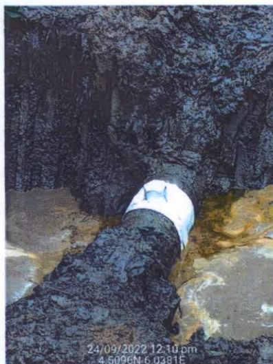
FIG 2-3: Incident Facility repaired and Aqua wrapped
